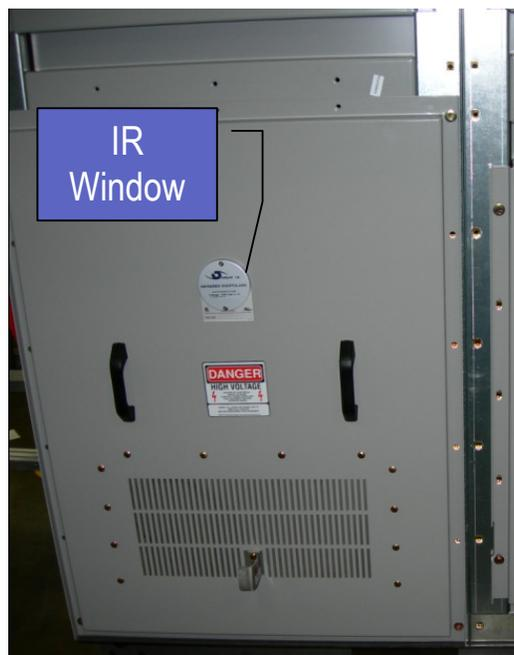
**Figure 2. IR-transparent windows for manual inspection of the temperature.**
