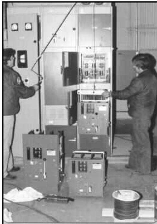
These technicians are removing some large air drawout circuit breakers from their cubicles for testing and servicing. Regular maintenance should be scheduled and electrical testing should be performed to ensure reliability of the electrical protection system.
