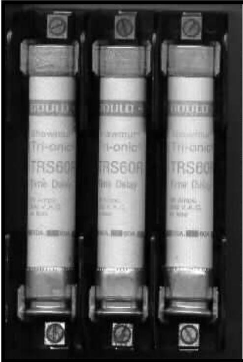
Fuses such as these provide inexpensive and reliable protection from catastrophic failures and extreme fault currents.
